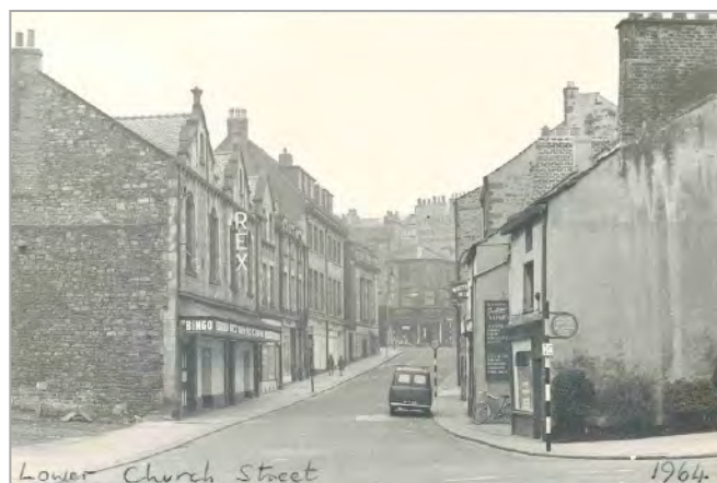
Figure 69: Lower Church Street in 1964. No. 2 appears to be an early C18 building which, like grade II listed no. 6, had a very large gable chimney stack, since removed. St Nic's has replaced most of the buildings on the left-hand side of the road (Lancaster City Museums).
