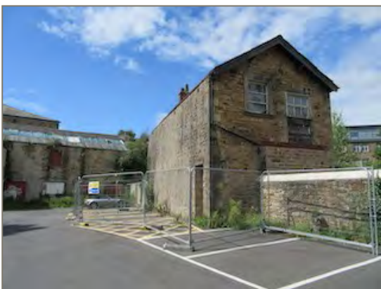
Figure 81: C19 former workshop building, St Leonard's Place
