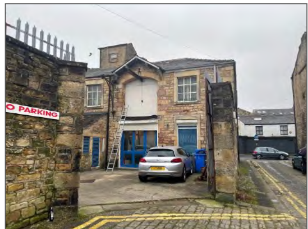
Figure 52: Welch's former grocery warehouse, Nile Street
