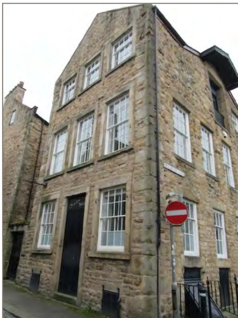
Figure 31: Late C18 warehouse to the rear of 11 Chapel Street.
