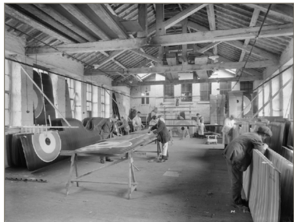
Figure 20: The production and inspection of bi-plane wings at Waring and Gillows, Lancaster, 1917 [Historic England ref. BL23741/036], thought to be in the 'Old Mill' on North Road.
