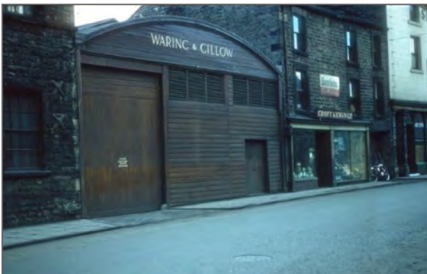
Figure 21: Waring & Gillow 1919 hangar-style building, photographed c.1960
