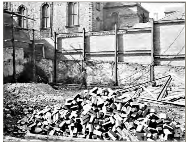
Figure 85: The cleared Phoenix Foundry site during the 1930s, looking towards the former Centenary Chapel & School (previously the Lawson Mansion), by this time it formed part of the Drill Hall (credit Susan Kennedy, Lancaster Past & Present)
