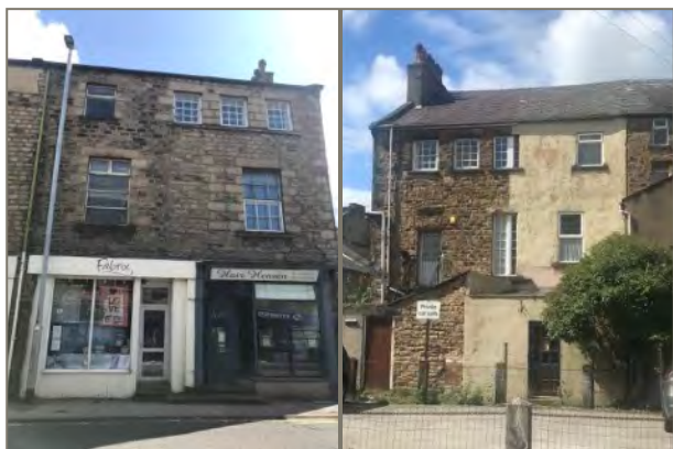
Figure 48: No.s 37 and 39 North Road (front and rear) originally one house.
