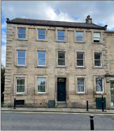
Figure 75: No. 127 St Leonard's Gate (grade II), the former Tramway, now student flats
