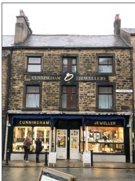
Figure 58: 2-4 Damside Street, the former Dye House has been Cunninghams, a jewellers, since the late C19.
