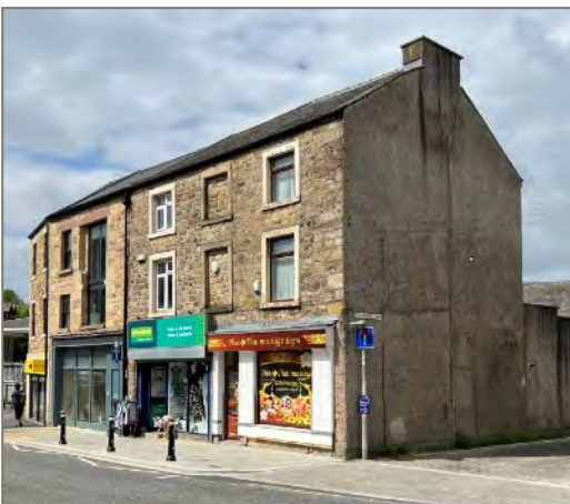
Figure 33: No. 10-16 Damside Street, on the site of the town's former mill, over the mill race
