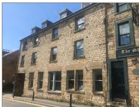
Figure 30: 98 St Leonard's Gate, a late C18 workshop building used by a series of coach builders throughout the C19, now student accommodation
