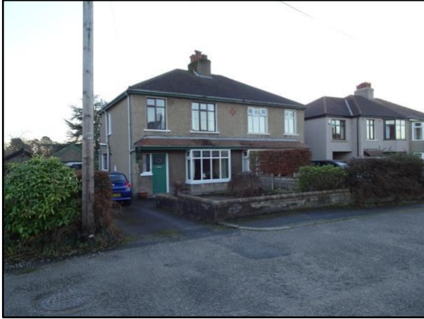
Photo 13. Semi-detached Houses on Kirklands
