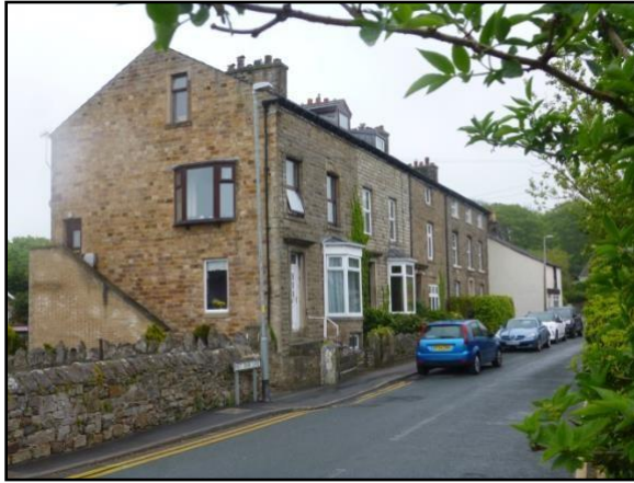
Photo 7. Georgian Terrace, Hest Bank Lane
