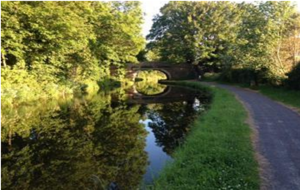
Photo 4. Hatlex Bridge (No. 119) on Lancaster Canal
