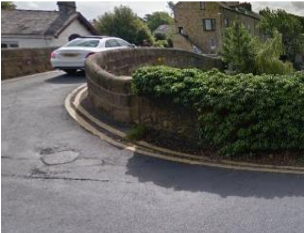
Photo 33. Canal Bridge on Hest Bank Lane
