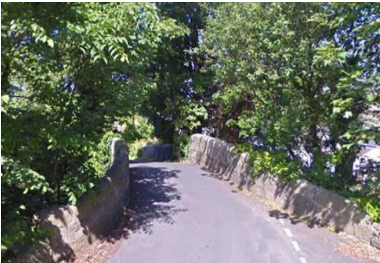
Photo 34. Canal Bridge on Hatlex
