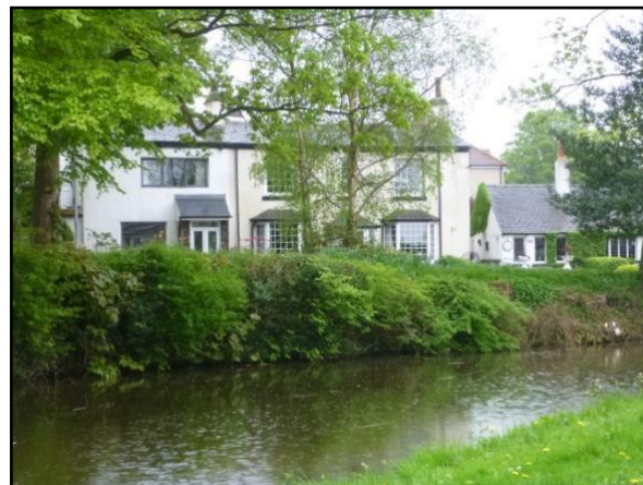
Photo 9. Terrace houses by the canal on Hatlex Lane
