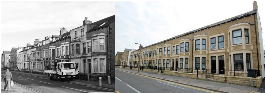
Photograph of Westminster Road before and after refurbishment
